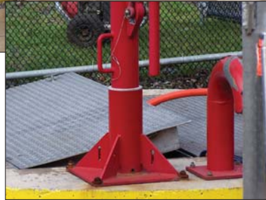
Above, the Gamajet system operates inside a wet well. Right, the hose connected to the cleaning tool passes beneath the wet well cover.
